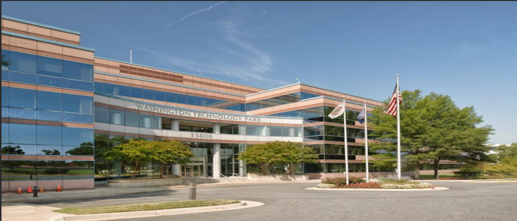
UNICOM Technology Park (UTP -- Washington DC)
